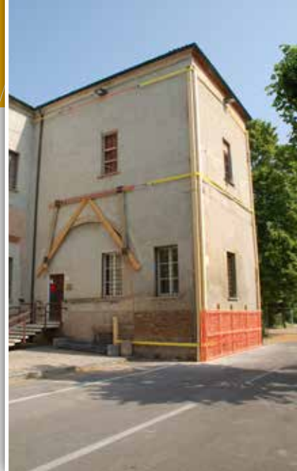
The provisional strengthening of the "Ala Giorgi"
