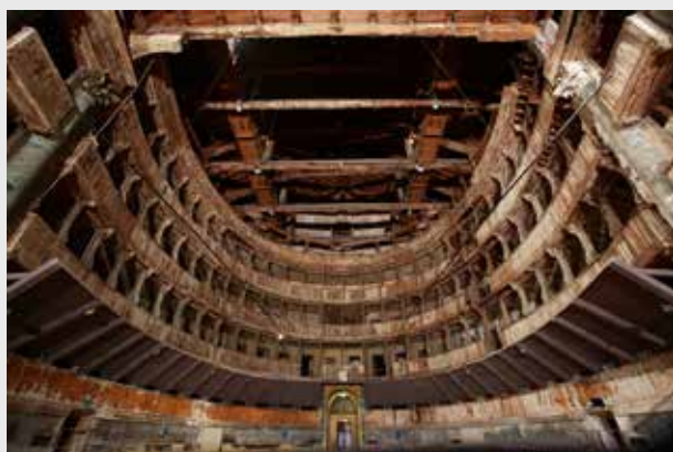
The main hall of the theater and the wooden parapet of the boxes before the beginning of the restoration. The advanced state of degradation can easily be noticed.
