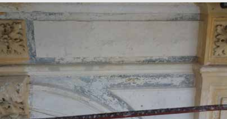
Stratigraphic research lead on the external façade; the original colors were white and grey instead of the yellow-brown palette
