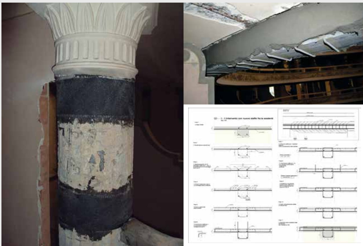
The reinforcement of the columns and of the existing concrete structure
