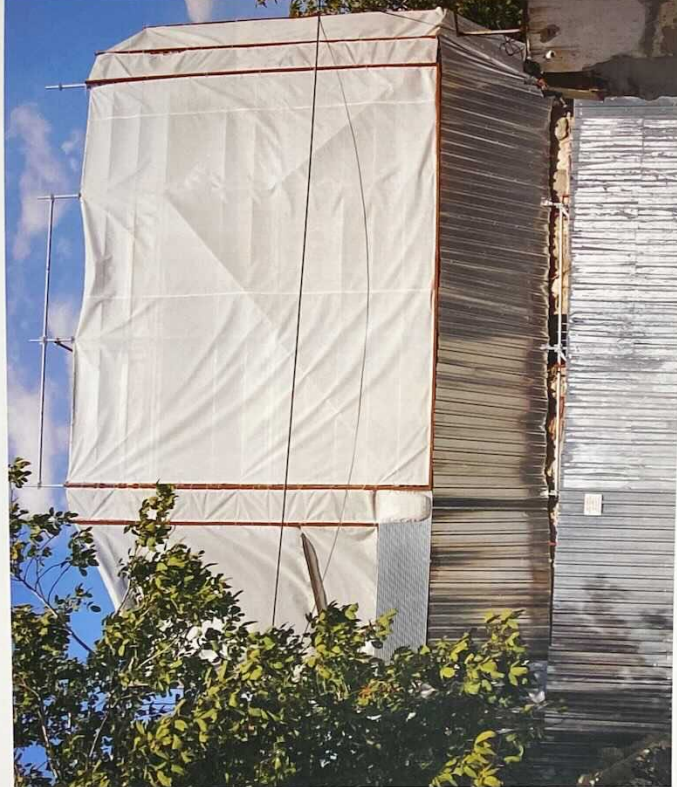
Figure 12. View of scarf-folding of the masjid.
