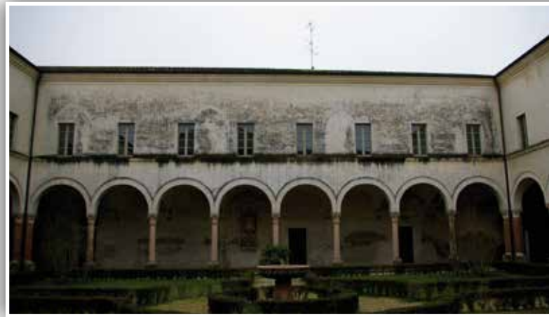
The northern façade of the Cloister of Secolari before and after the restoration
